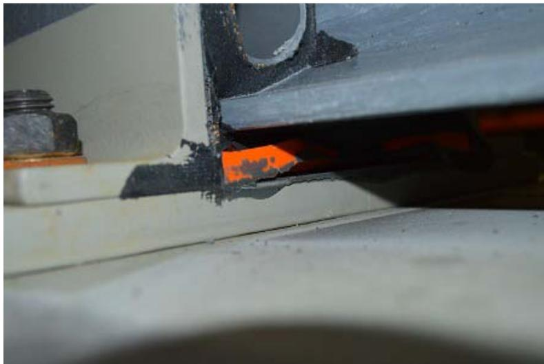
*Figure-5.51: Separation of Elastomer Strip from Steel Girder (Rear end)*
