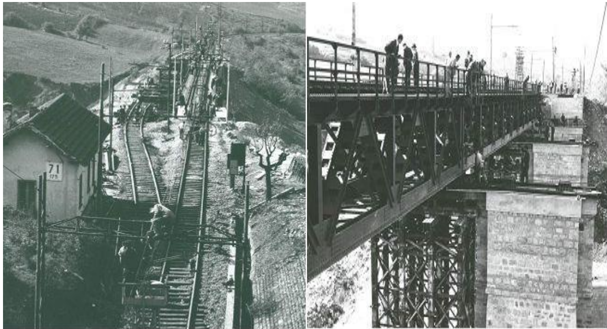
Figure 3.1: the bridge over the river Gesso after reconstruction
