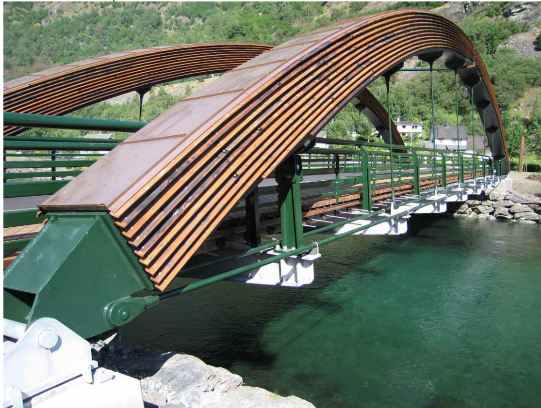
Fretheim bridge, Norway
