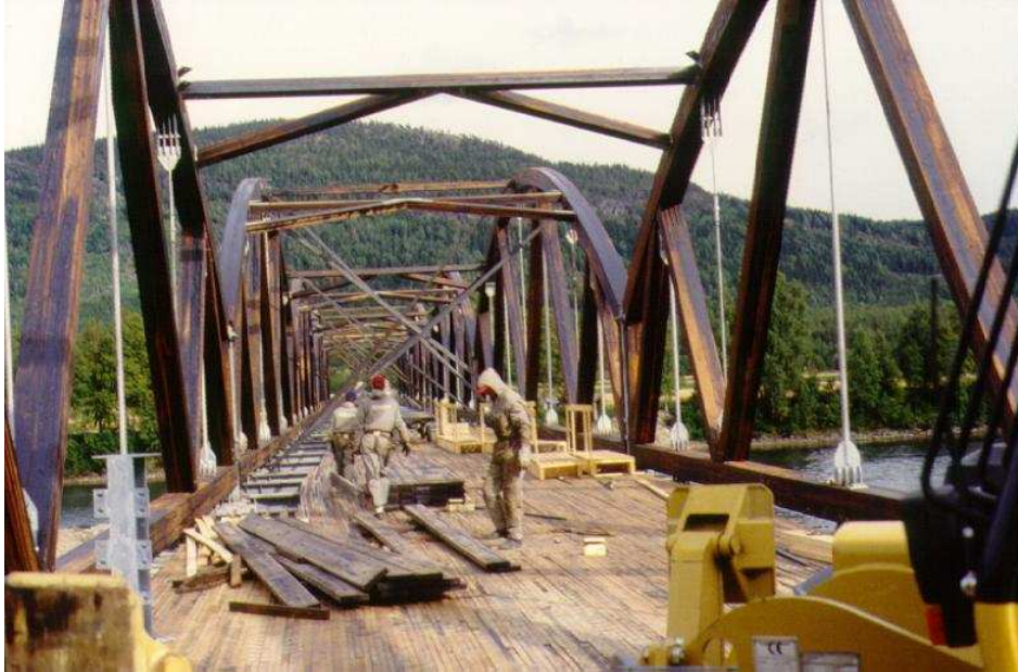
Evenstad bridge, Norway
